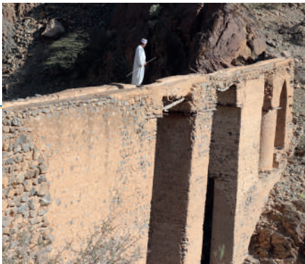
Canal-bridge to allow water overtaking a depression in a valley ( wadi bani kharous ). © University of Nizwra.
